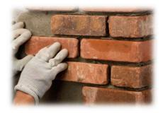
Then continue up the corner with a 110mm cut brick facing or corner piece with the same application technique.
