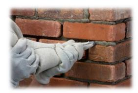
Put down some dropsheets around the job and with the mix now ready simply fill the joints. There is no "right" way to do this, it's just a matter of perseverance & keeping the wall as clean as you can.
